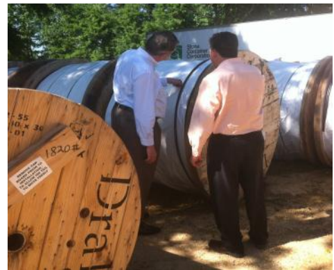
A NTIA Federal Program Officer visits Contact Network in Jackson, Mississippi, discussing the cable staged for installation along the route of a BTOP-funded fiber-optic network.
